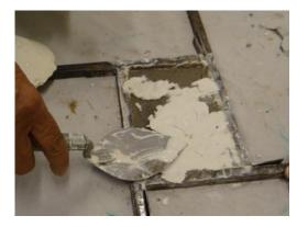
**Second Layer:** Even this layer is composed of lime and marble powder in the same proportions but the marble powder should be finer. When it is semi-dry the third and final layer should be applied.
